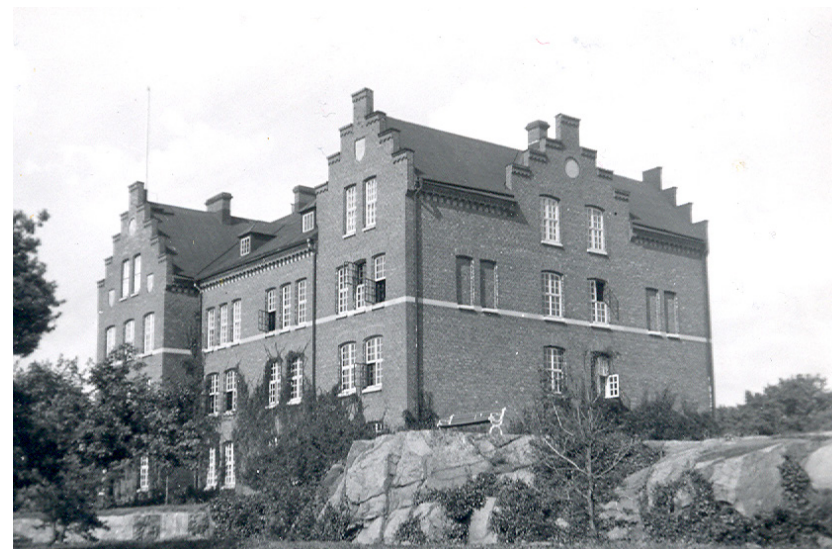
The joint services collection station in Karlskrona.
